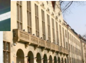
Main building (A-1)
